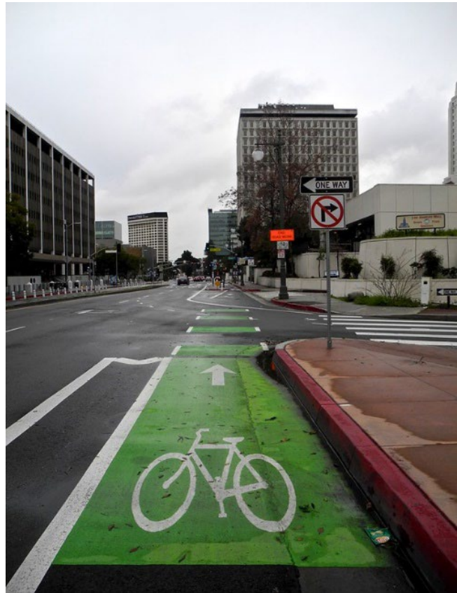
Figure 5-7. Example bike lane markings at an intersection where right turns are not permitted
