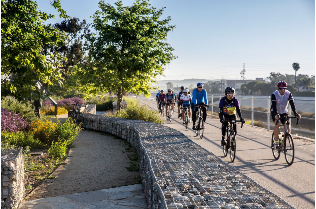
Figure 10-13. Low gabion wall barrier and seating
